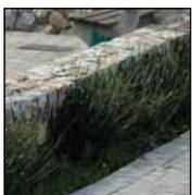
In-situ natural sandstone wall with concrete capping
