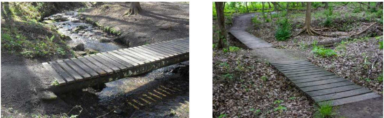
Figure 21. Bridges and boardwalks
