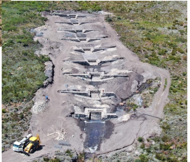
Figure 58 The weirs being constructed in 2021
