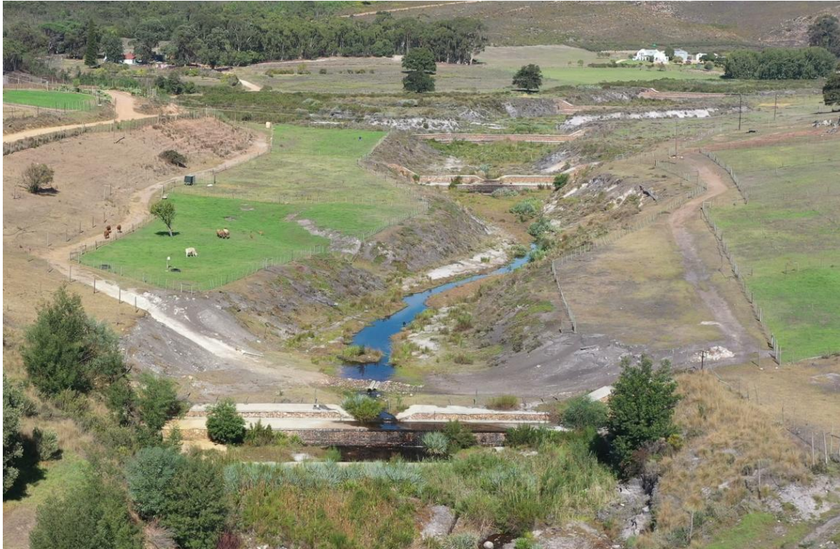
Figure 57 The gulley with a cascade of 5 weirs today
