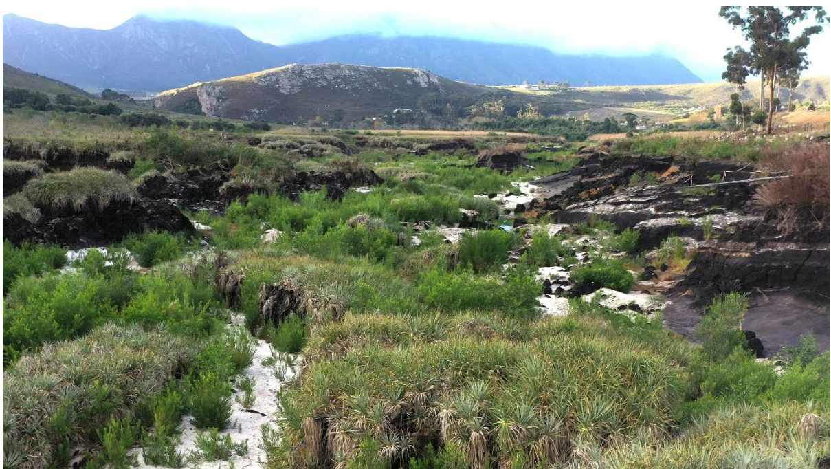
Figure 5 Looking upstream over where the headcut had been in August 2023. The gully is now about five times wider and several meters deeper.
