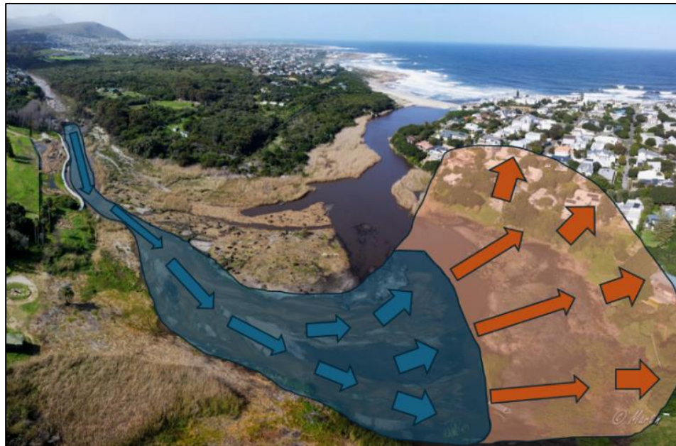
Figure 3.11. Blue: movement of sediment and floodwaters into the estuary during the September 2023 floods. Orange: anticipated flooding and sediment deposition within the Town of Onrus during future flood events should current conditions persist.
