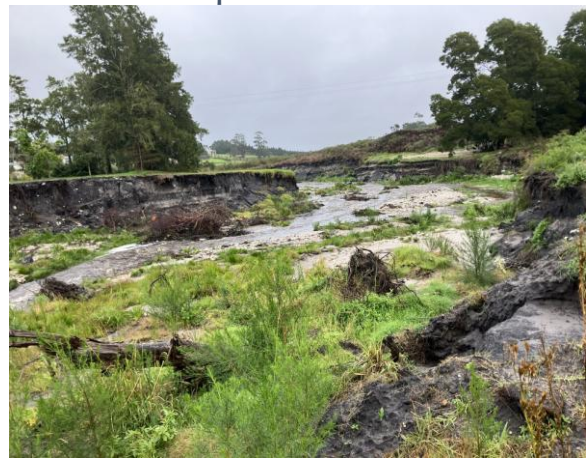
Photo 3D Large, low-lying culverts in the Onrus River (upper reaches) create concentrated flows into the downstream system, triggering channel incision and resultant loss of valley bottom wetlands, including possible peatlands
