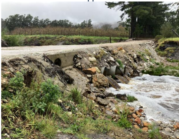
Photo 3D Large, low-lying culverts in the Onrus River (upper reaches) create concentrated flows into the downstream system, triggering channel incision and resultant loss of valley bottom wetlands, including possible peatlands
