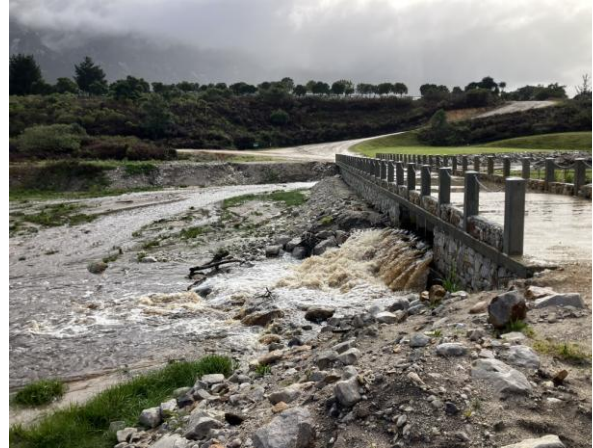
Photo 3F Downstream view of Onrus River, with concentrated flows through narrow culverts that precipitate downstream erosion and channel incision
