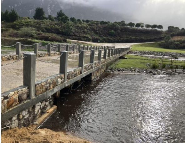
Photo 3E Upstream view of Onrus River, being entrained through narrow culvert
