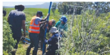
Installing a deep piezometer (Photo: AT Grundling)
