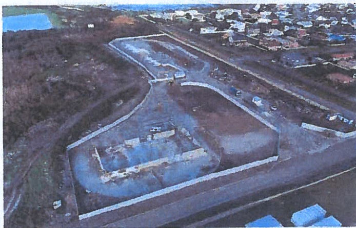
After a three-month delay due to damage caused to the steel structure of the new materials recovery facility building by strong winds in March, construction is back on track and expected to be completed by the end of August.
