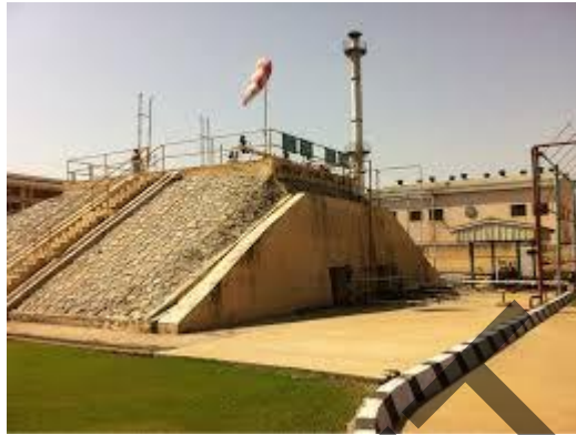
Example of a mounded tank facility
