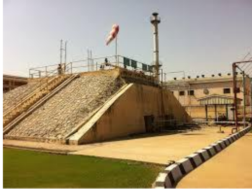
Example of a mounded tank facility
