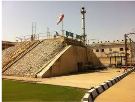
Example of a mounded tank facility
