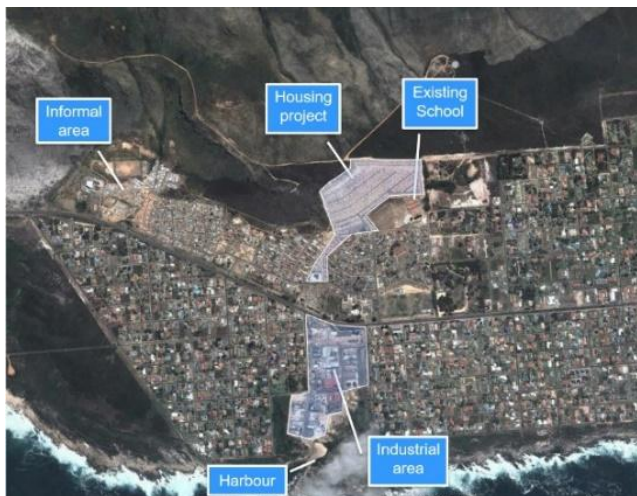
Figure 17: Kleinmond integrated housing development
