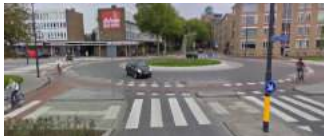
IMAGE 114. PEDESTRIAN FRIENDLY TRAFFIC ROUNDABOUT WITH PEDESTRIAN CROSSINGS ON ALL FOUR APPROACHES
