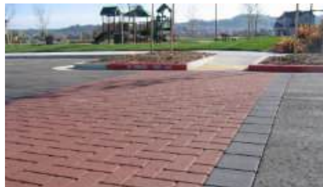
IMAGE 86. PAVED PEDESTRIAN CROSSING AND INTERSECTION
