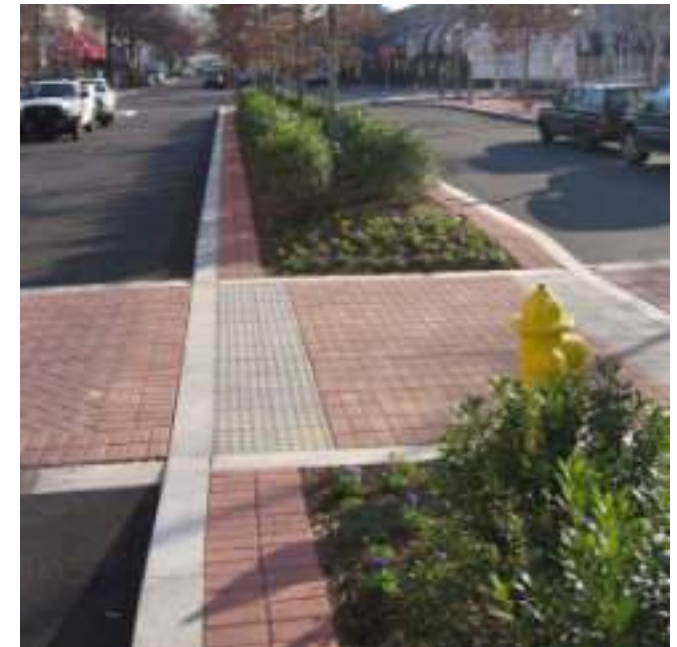
IMAGE 113. PAVED PEDESTRIAN CROSSING WITH MEDIAN TO REDUCE CROSSING LENGTH
