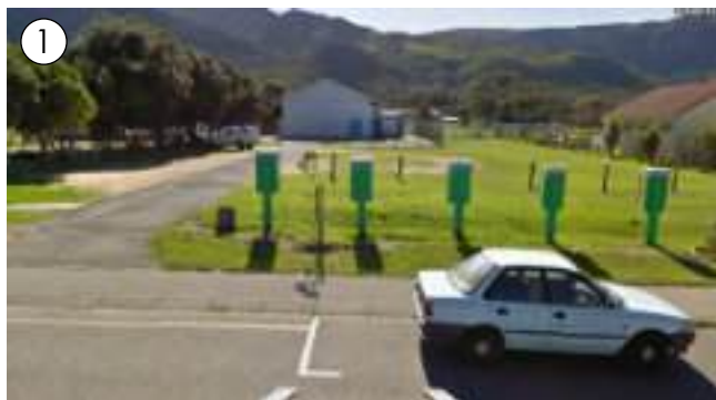
IMAGE 97. TELKOM SITE ON MAIN ROAD
