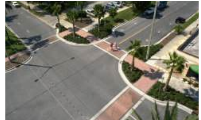
IMAGE 115. PAVED PEDESTRIAN CROSSING WITH KERB BUMP OUTS TO REDUCE CROSSING LENGTH
