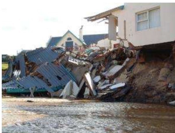
(c) Flood damage
