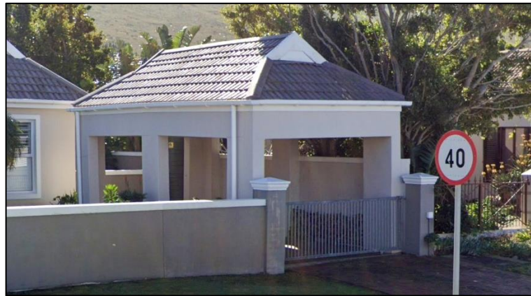
Figure 1: Photo of the existing carport
