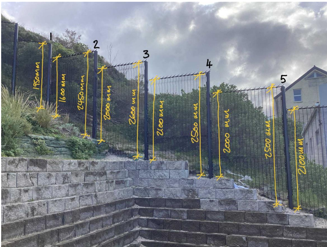
FENCING ON EAST BOUNDARY
