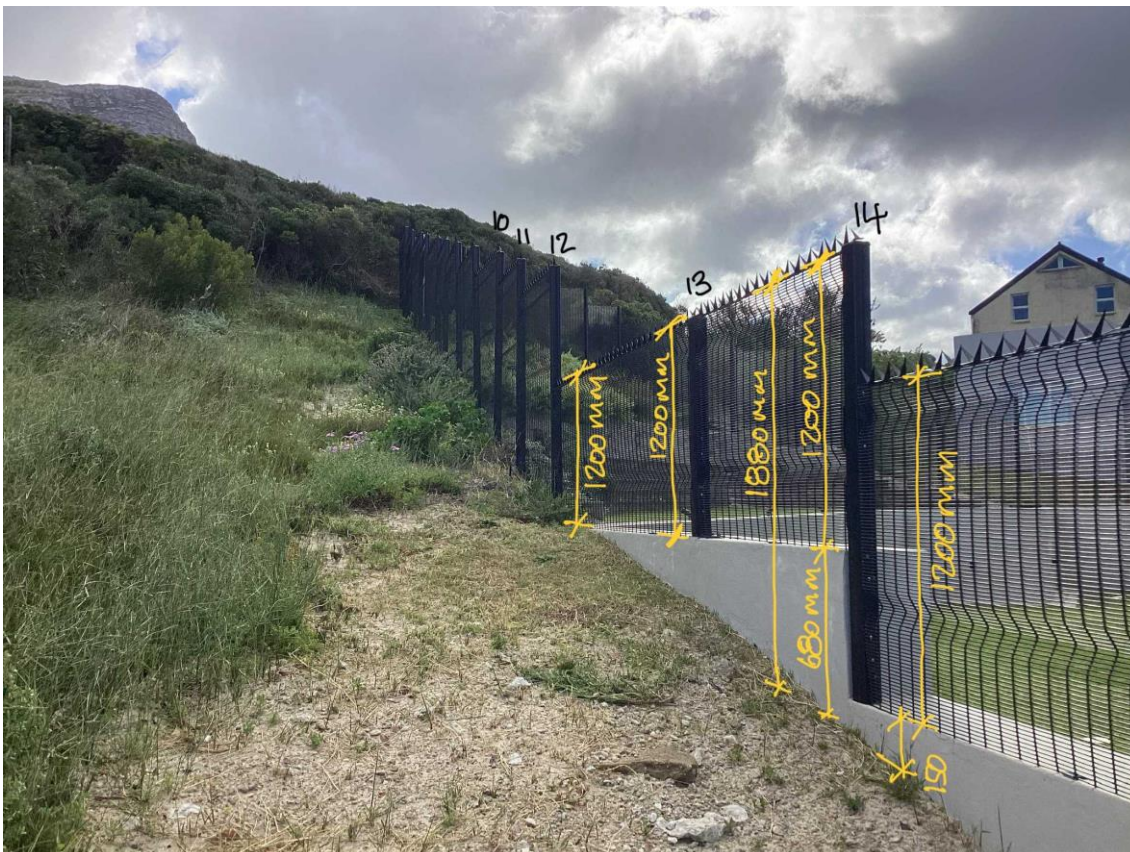
FENCING ON WEST BOUNDARY
