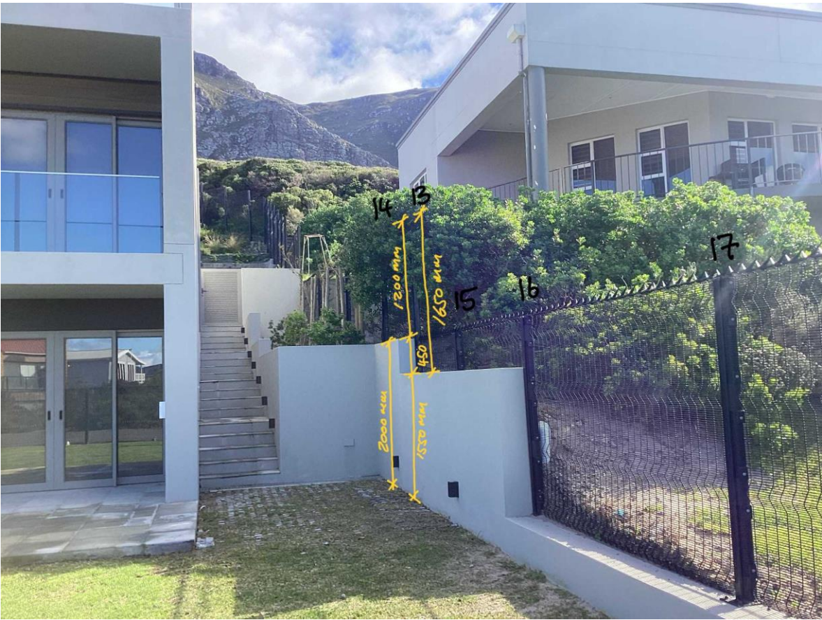
FENCING ON EAST BOUNDARY
