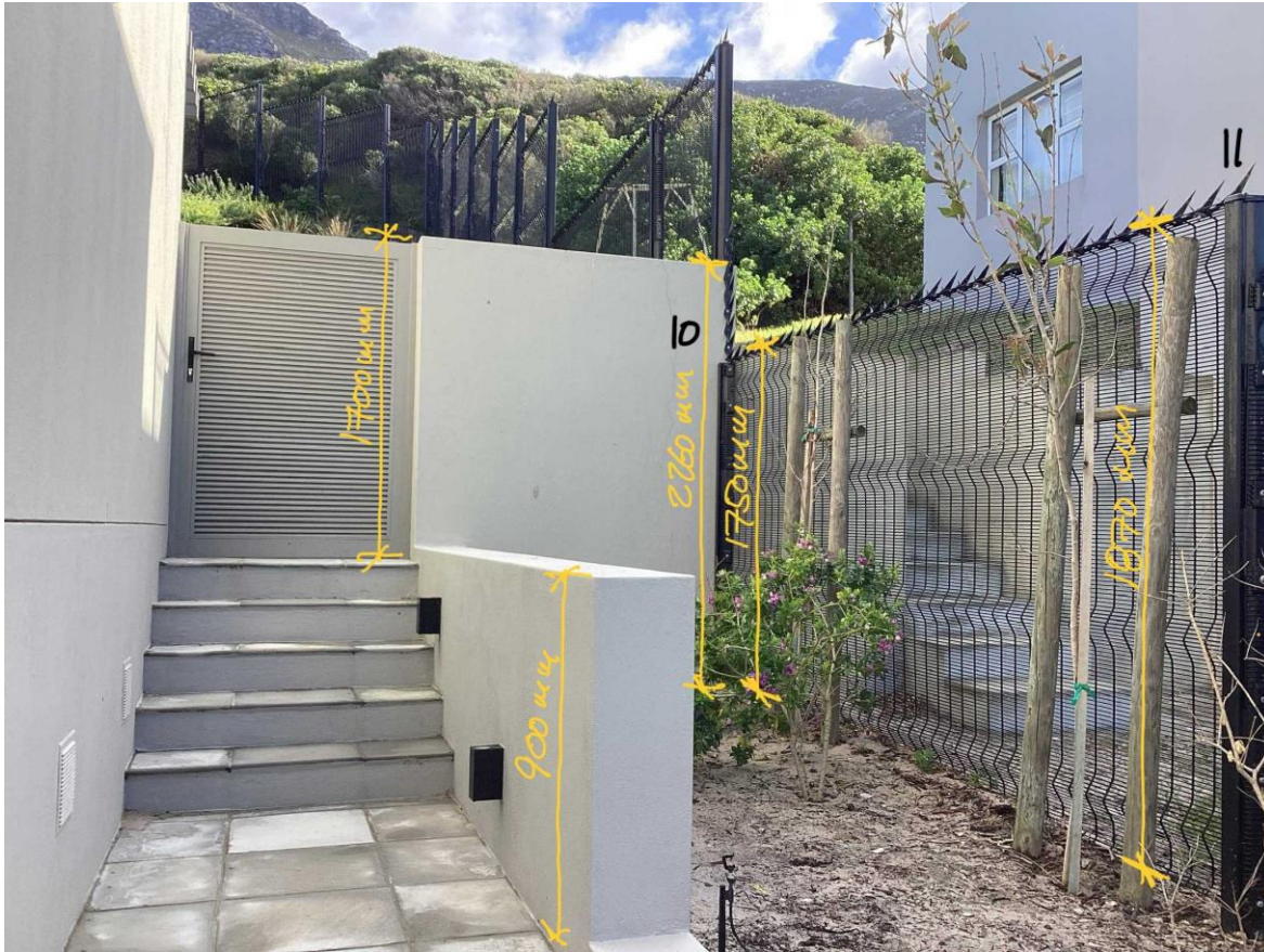
FENCING ON EAST BOUNDARY
