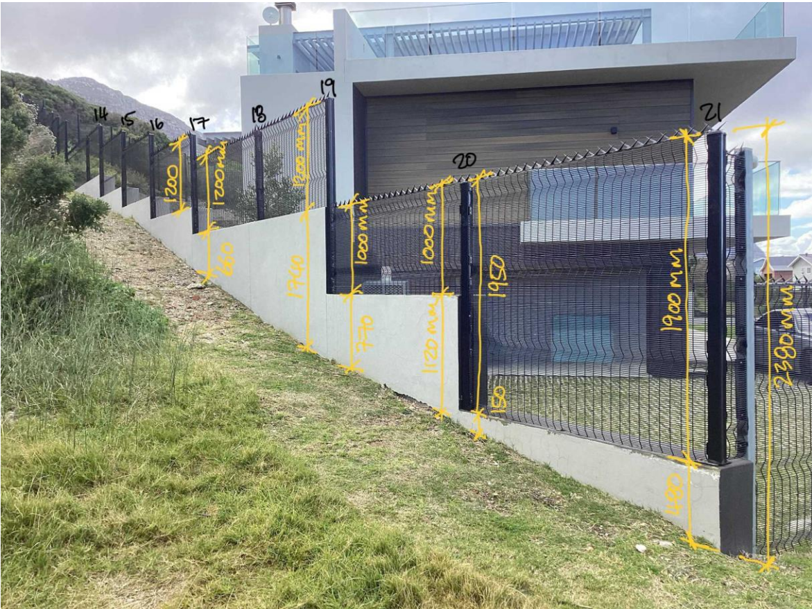
FENCING ON WEST BOUNDARY
