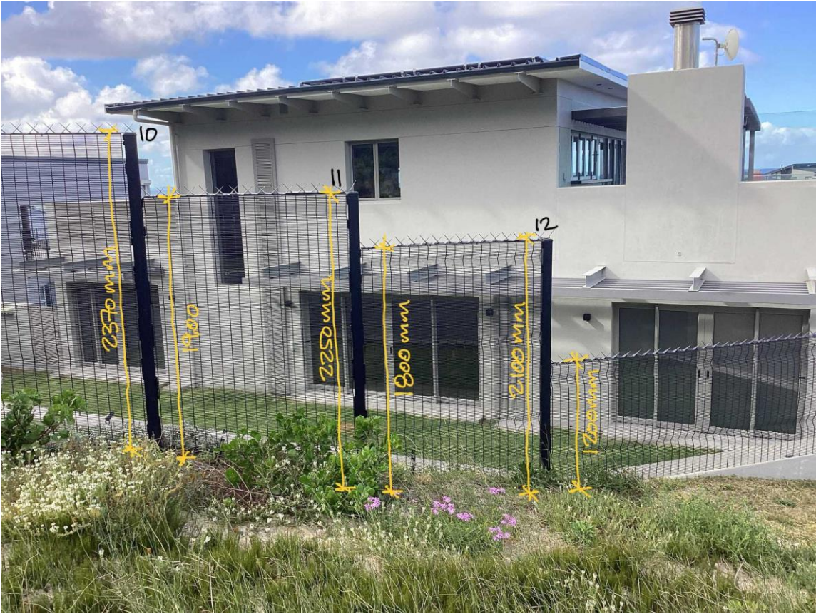
FENCING ON WEST BOUNDARY
