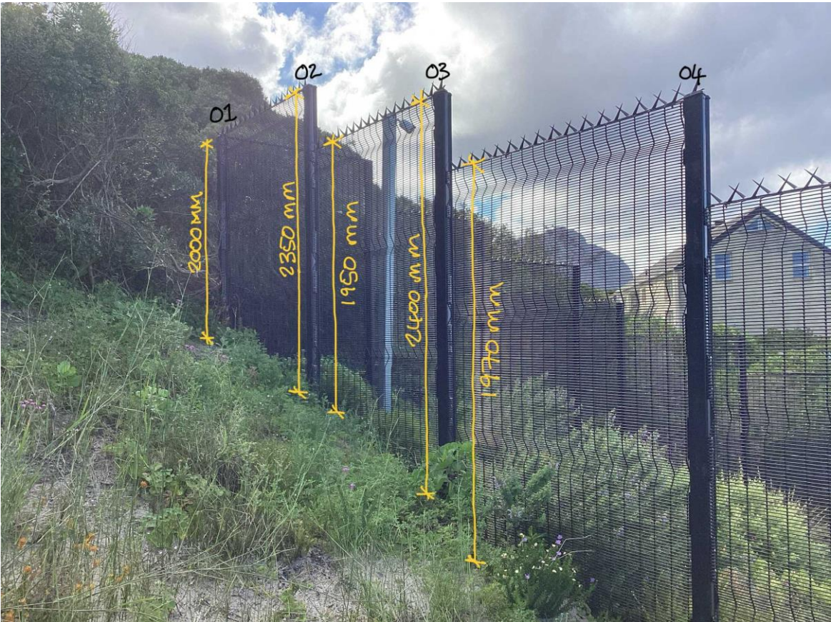
FENCING ON WEST BOUNDARY
