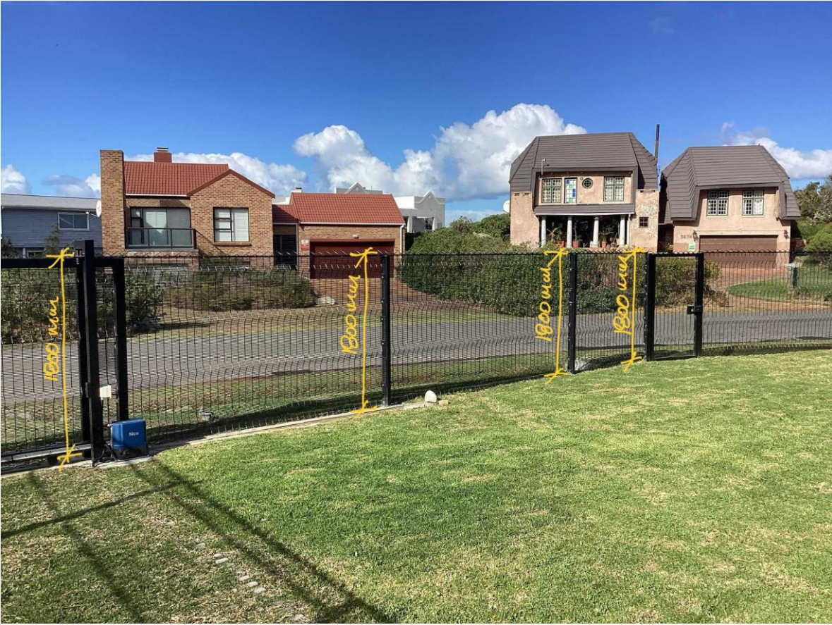
FENCING ON SOUTH BOUNDARY
