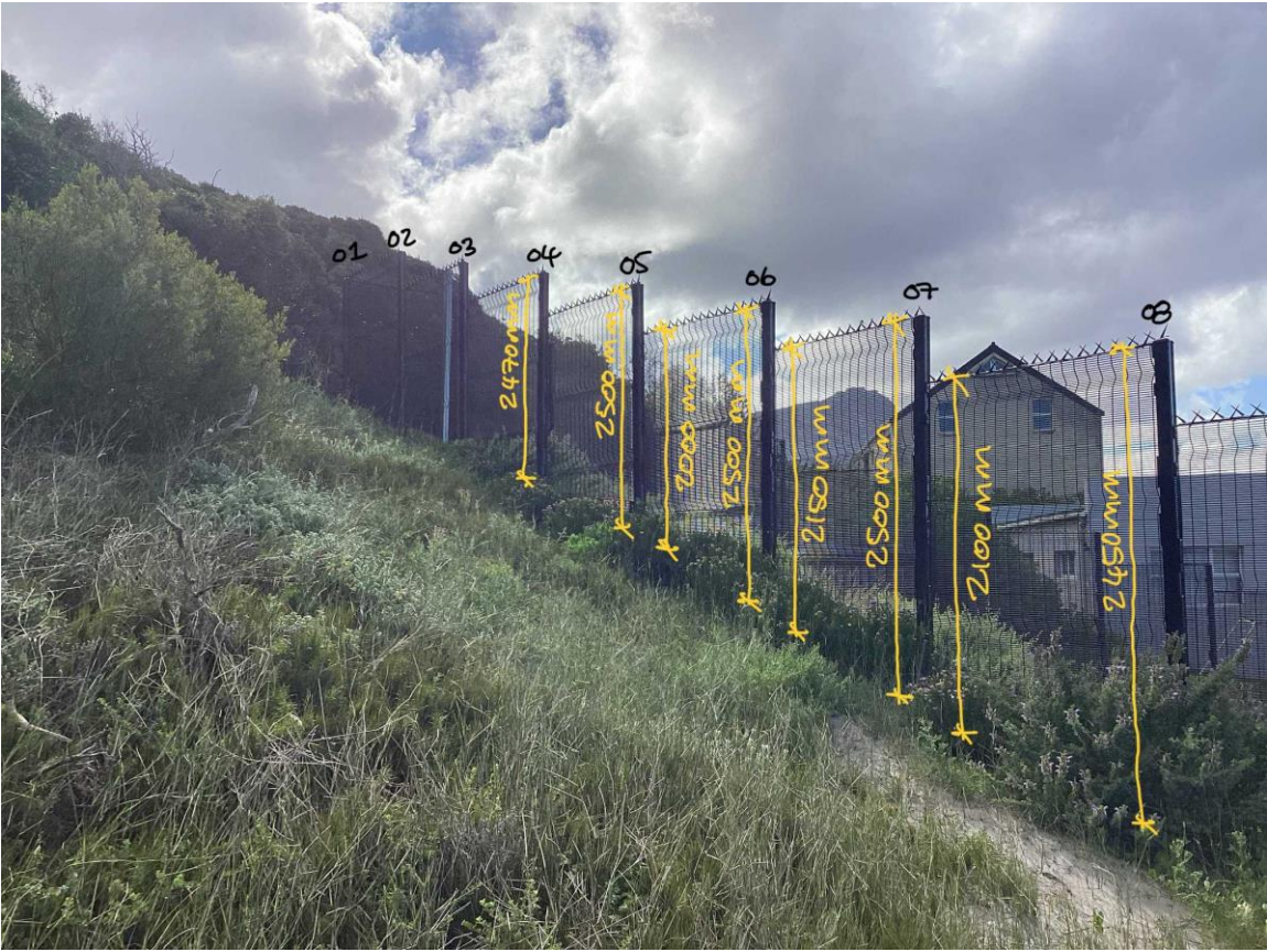
FENCING ON WEST BOUNDARY
