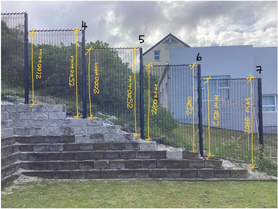
FENCING ON EAST BOUNDARY
