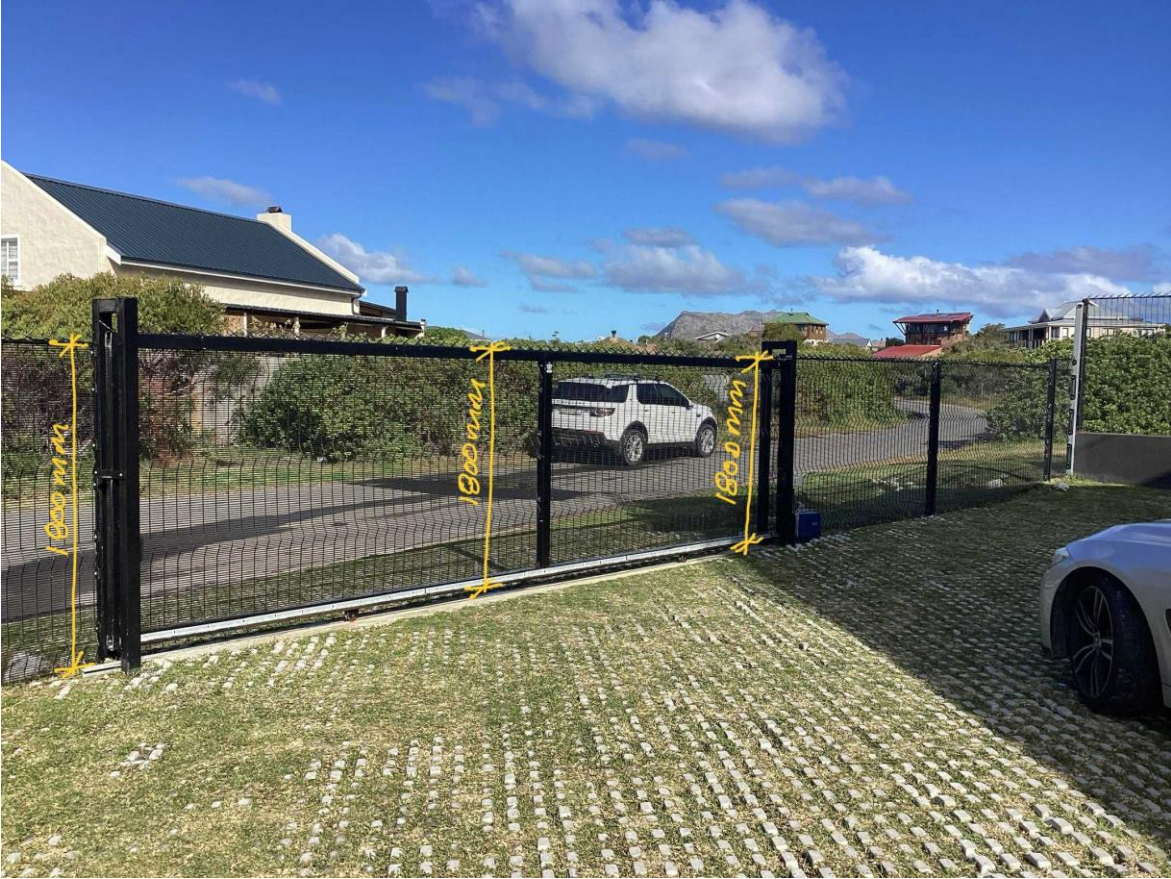
FENCING ON SOUTH BOUNDARY
