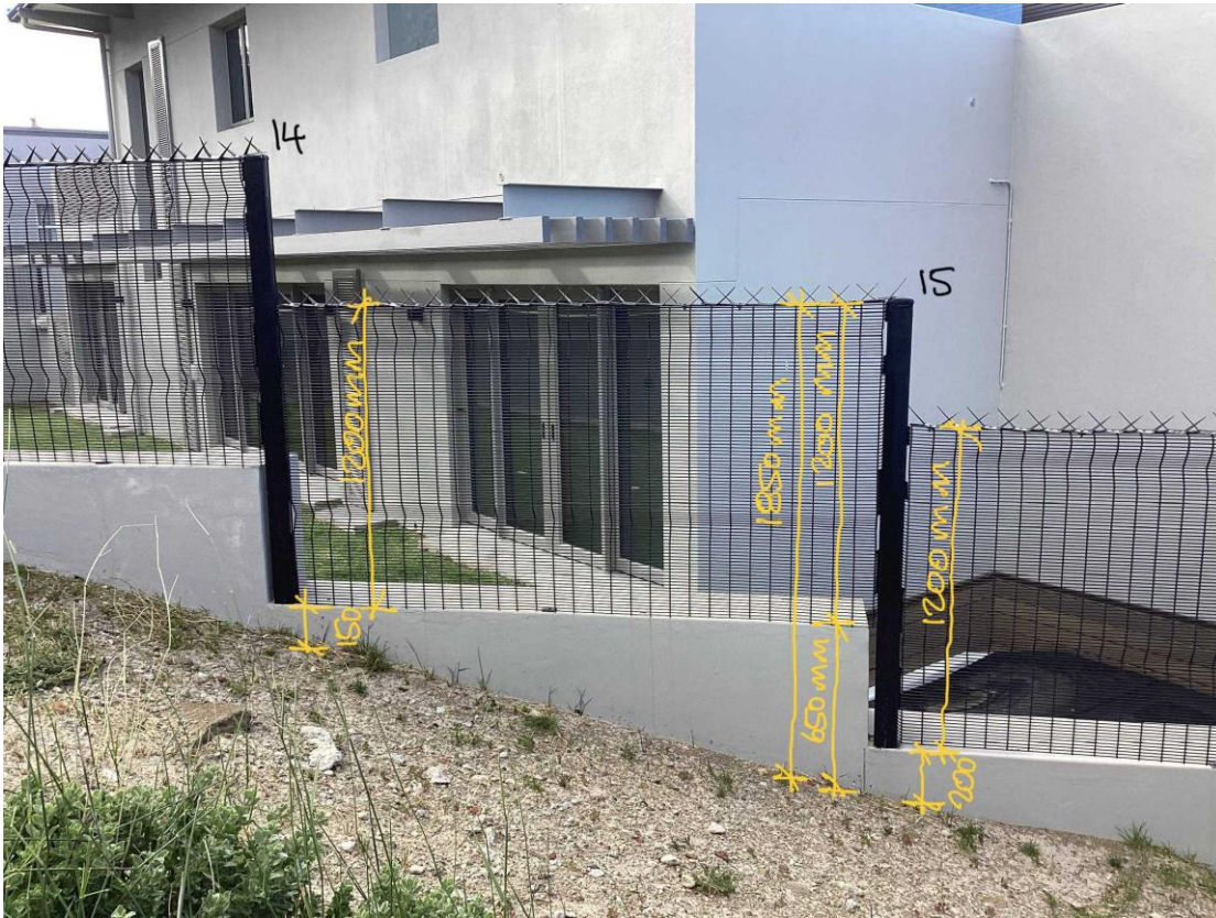
FENCING ON WEST BOUNDARY
