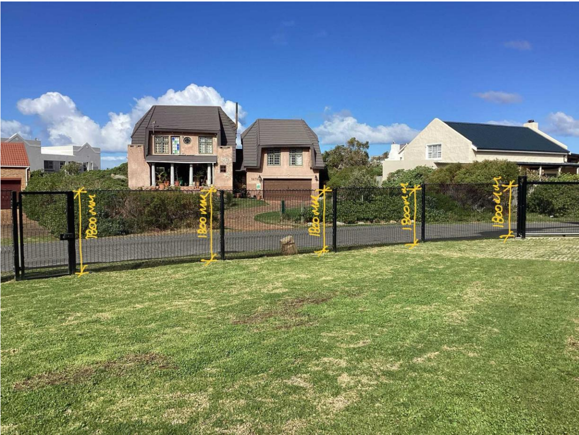
FENCING ON SOUTH BOUNDARY
