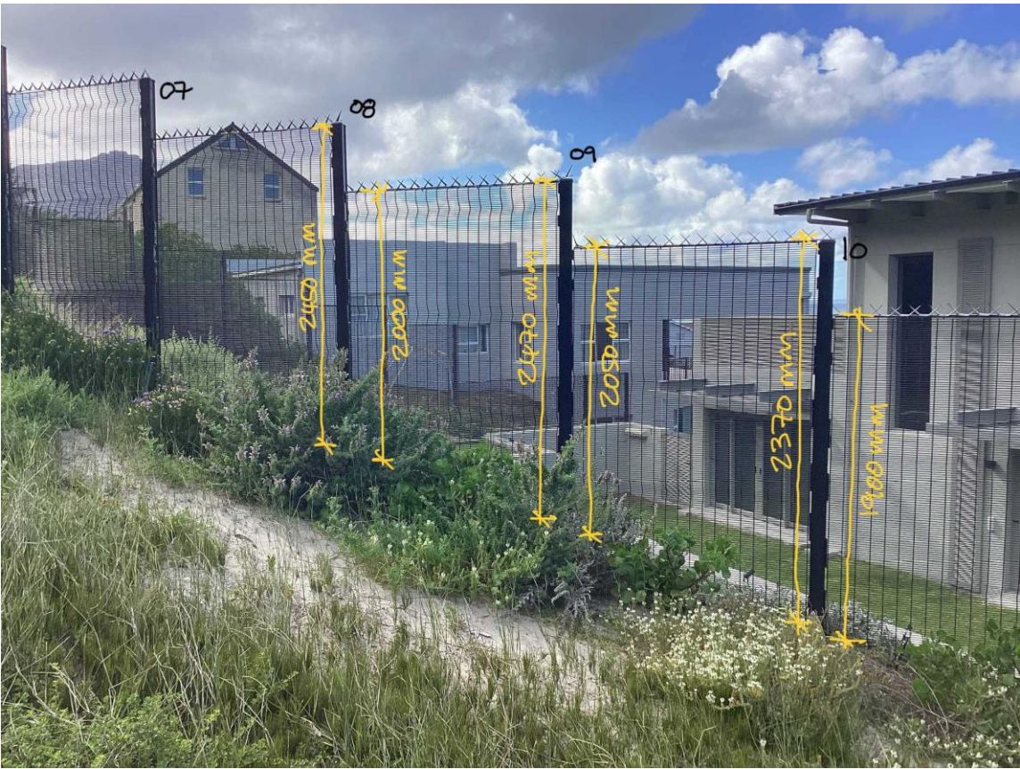
FENCING ON WEST BOUNDARY
