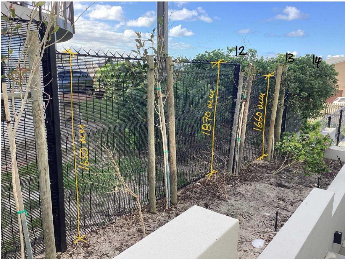
FENCING ON EAST BOUNDARY
