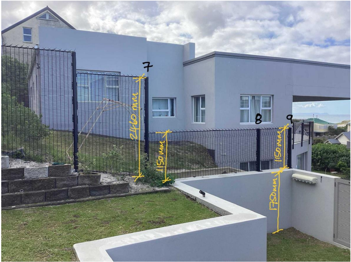
FENCING ON EAST BOUNDARY
