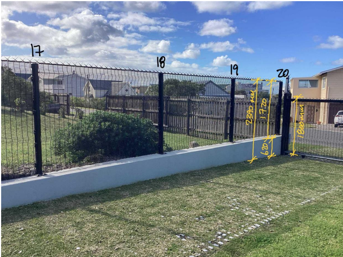
FENCING ON EAST BOUNDARY
