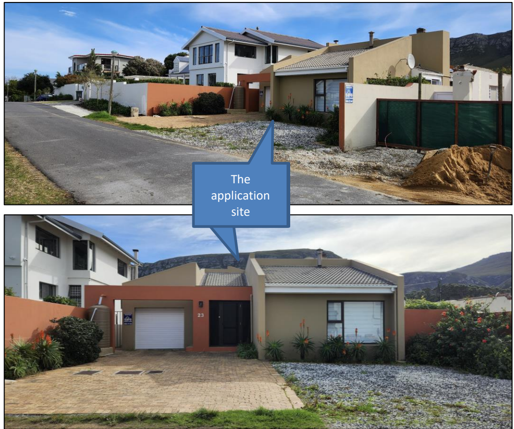
Figure 9: Photographs of the application area
