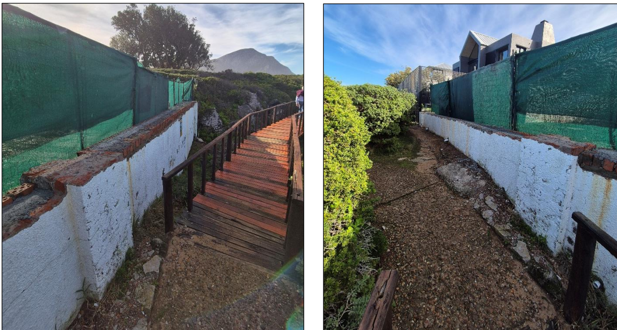
Figure 3: Existing retaining wall height
