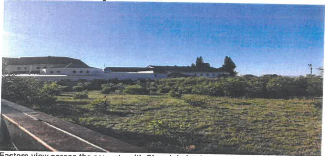
Eastern view across the property with Church in background
