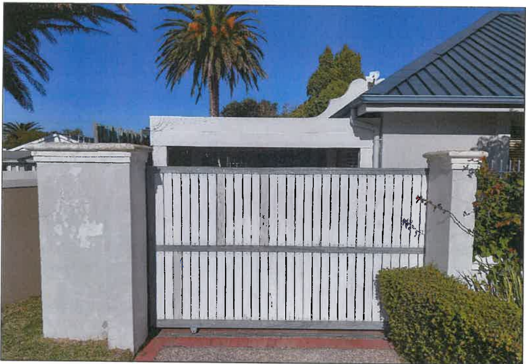
Figure 11: Photo of the carport
