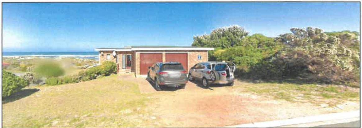
Figure 4 – Street view of the property from Vergesig Street
