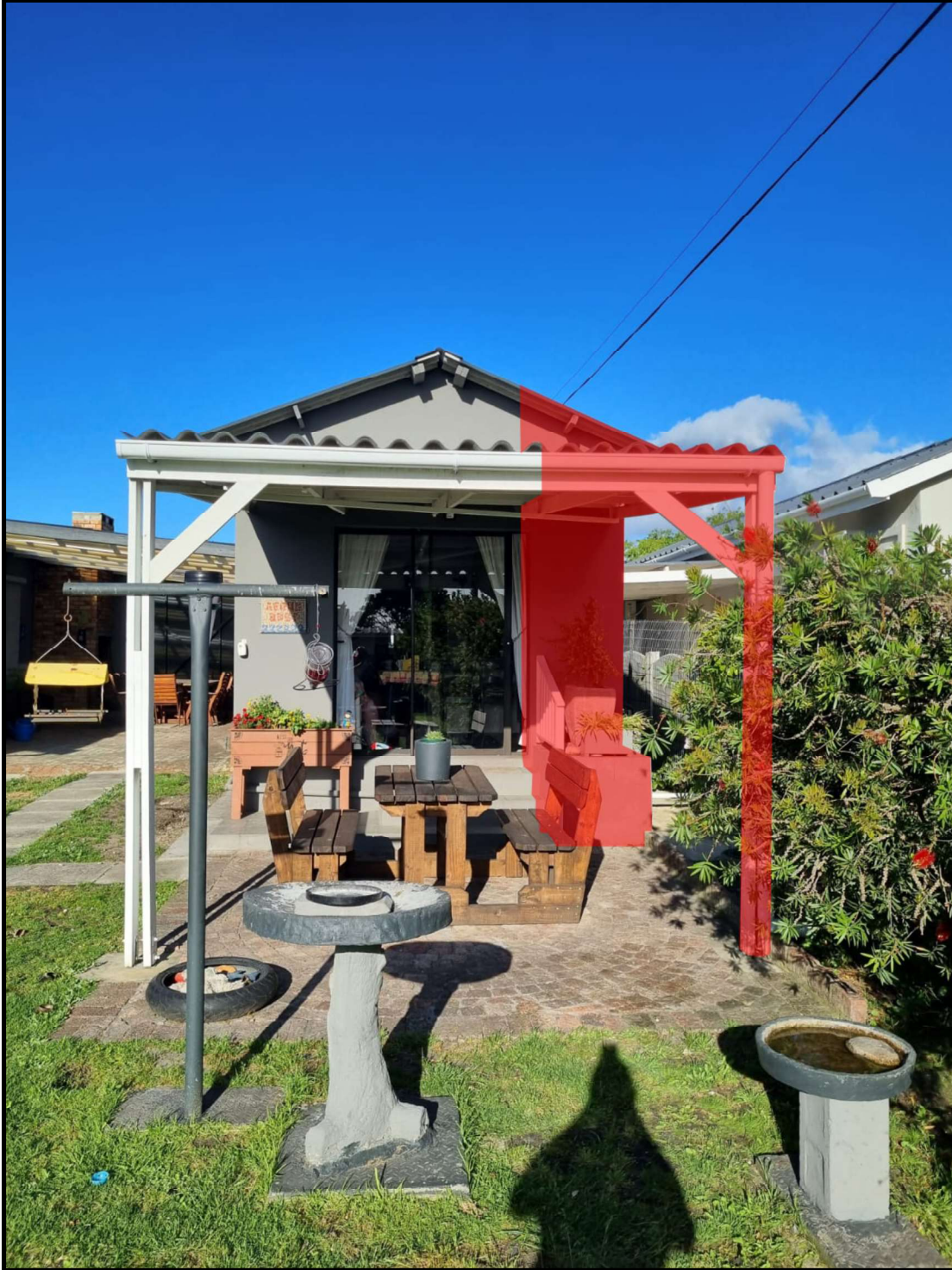
Second Dwelling and Covered Patio Exceeding Northern Building Line
