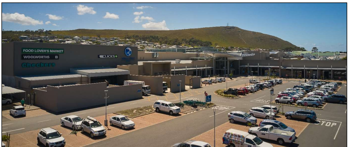
Figure 8 – The view of the shopping centre from the southern parking area.
