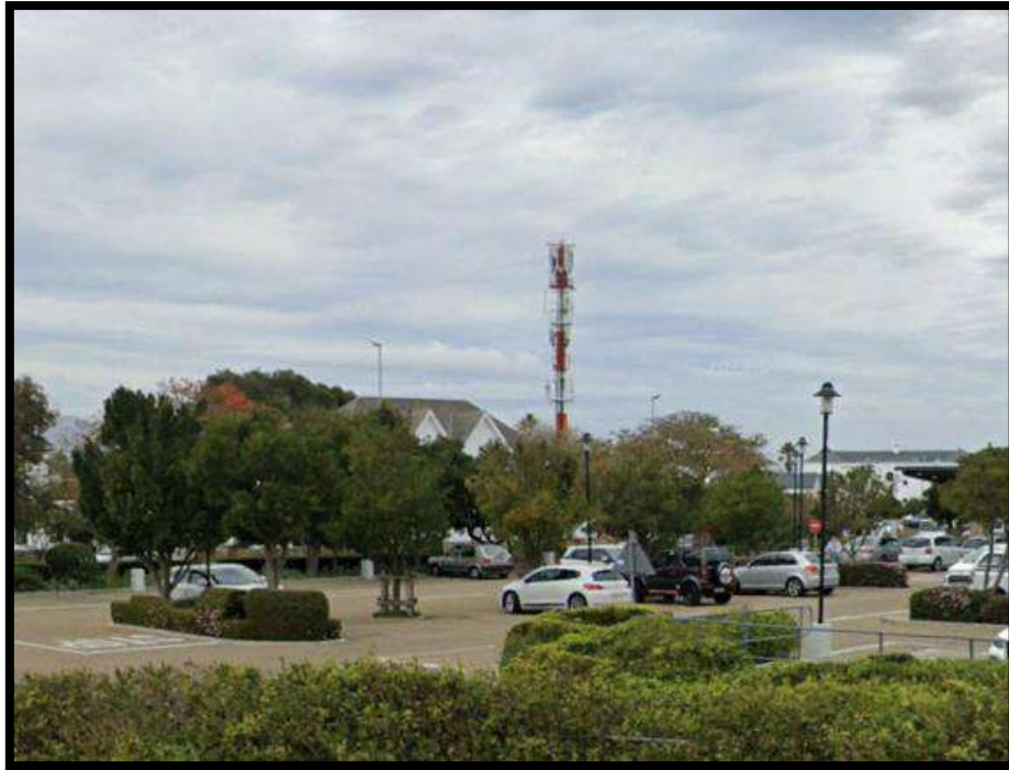
Figure 14 - Image of the Existing Transmission Apparatus from Royal Street
