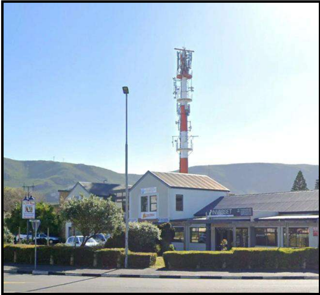
Figure 13 - Image of the Existing Transmission Apparatus from the circle in the Main Road
