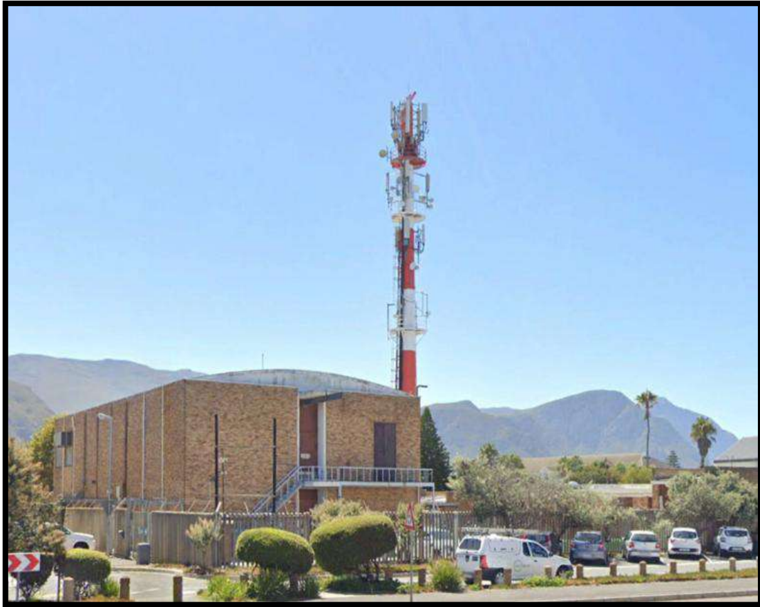
Figure 12 - Image of the Existing Transmission Apparatus from Mitchel Street
