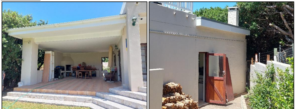
Figure 10: Photographs of the structures exceeding building lines.
