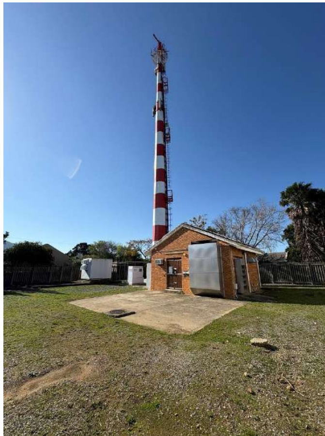
Figure 10 - Site Photo of Existing Transmission Apparatus
