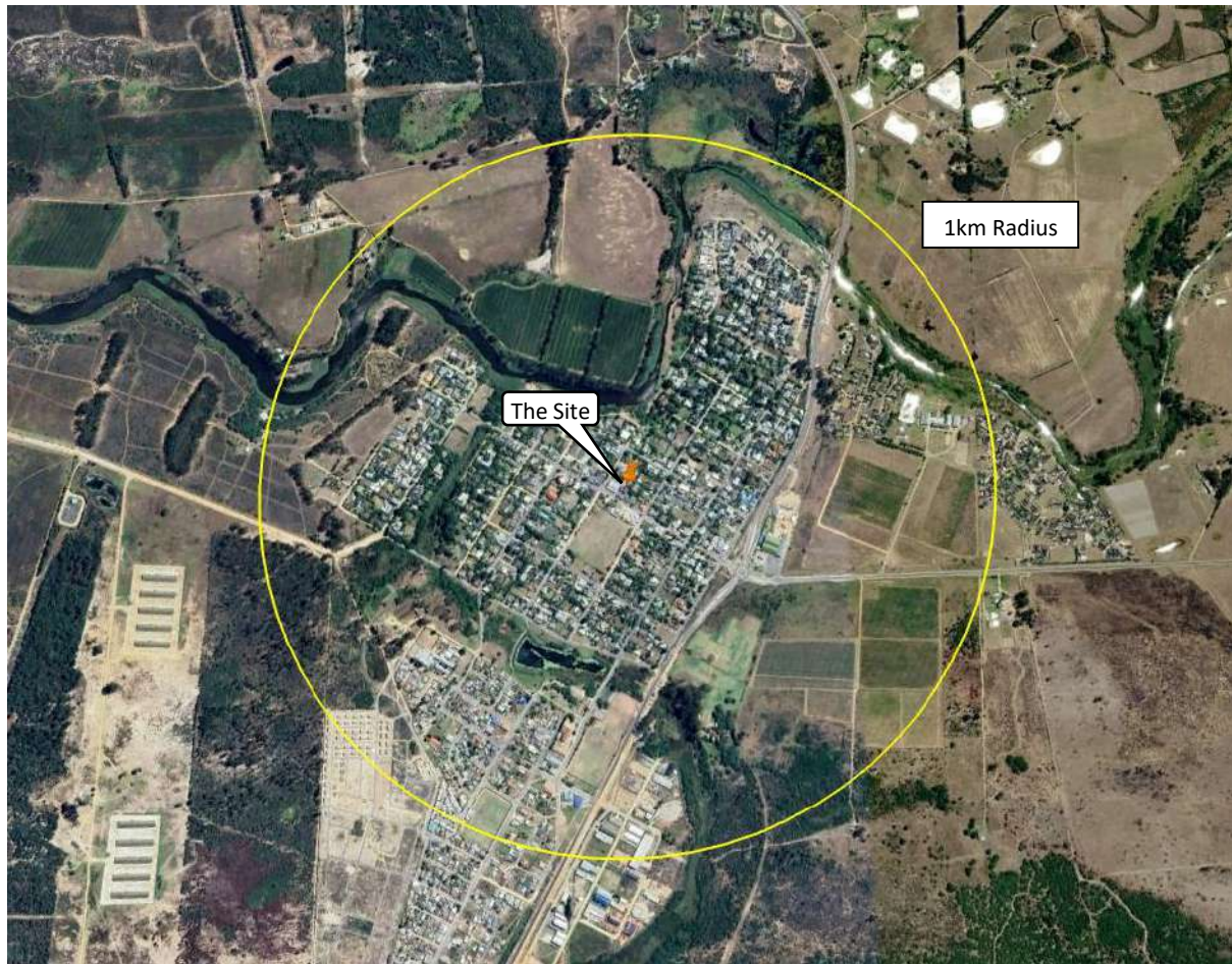
Figure 9 - Existing Transmission Apparatus in 1km of Existing Site
