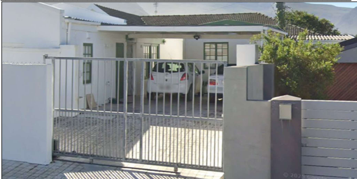
Figure 1: Existing Gardener's room and carport
