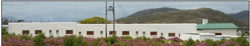
Main Building Eastern Elevation
