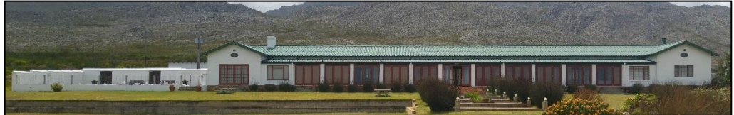
Main Building Northern Elevation
