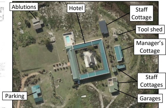
Figure 3: Existing lay-out of buildings to be used and converted for the development proposal
