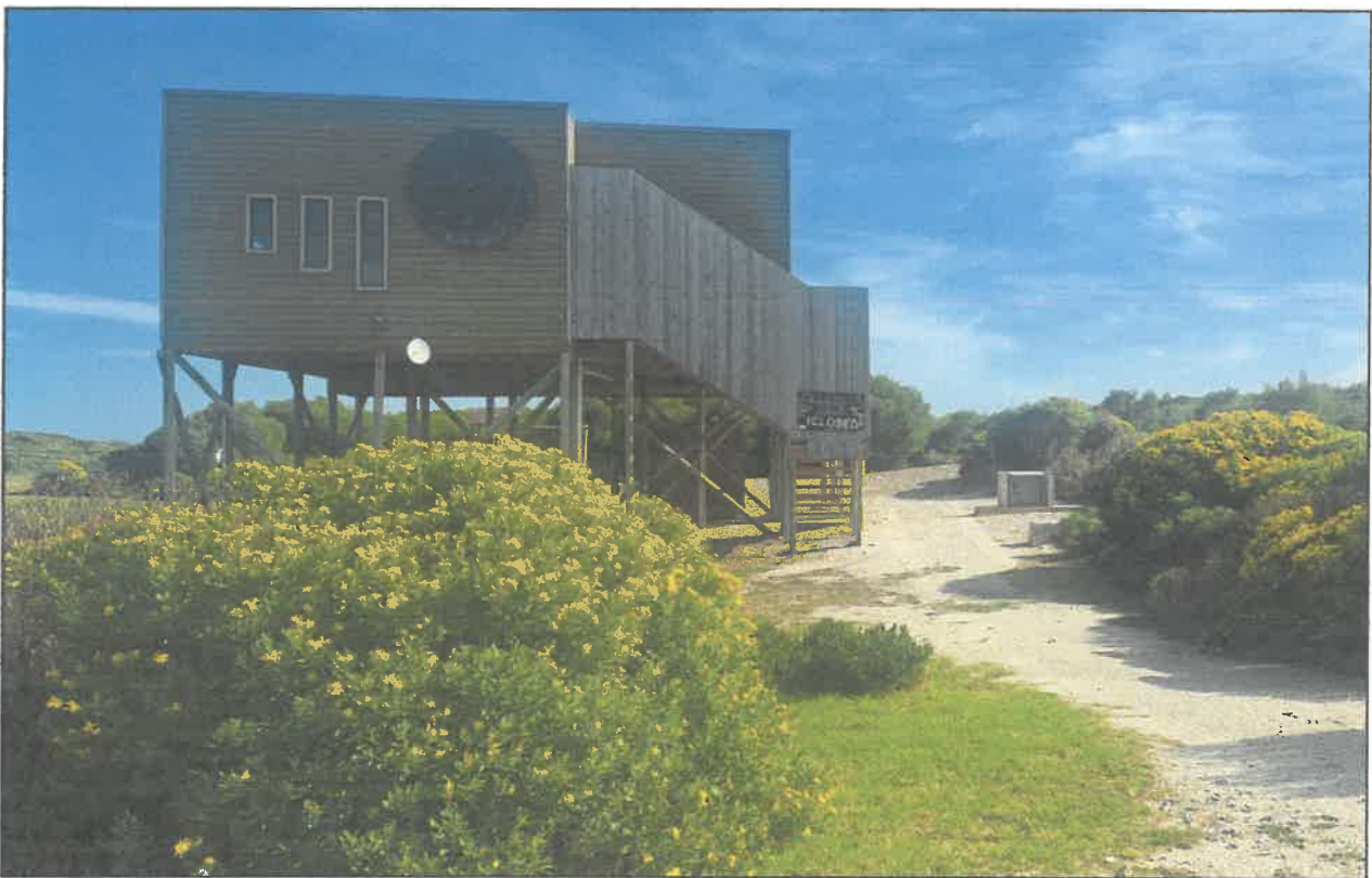
Photo of the existing building on Erf 329.
