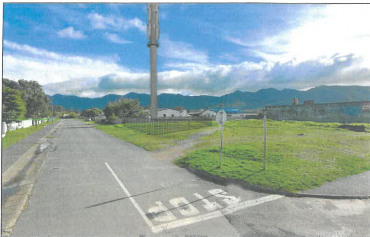
Figure 11 Illustration of mast at Poole street
