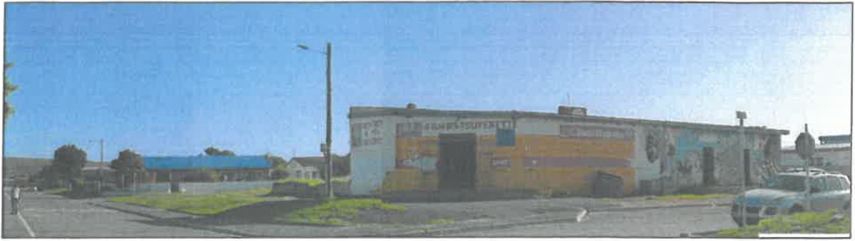
Photo 1 Superette site where mast to be installed
