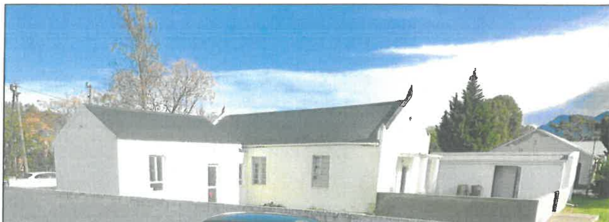
Photo 7 Historical church in Skool street, Erf 304
