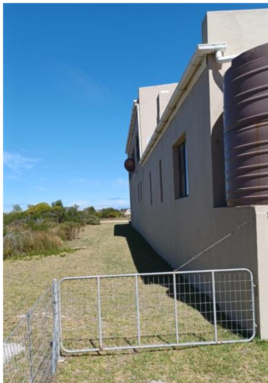
Image 1: As Built lounge and bedroom on first storey level and water tank positioned on the 2,085m eastern lateral building line.
