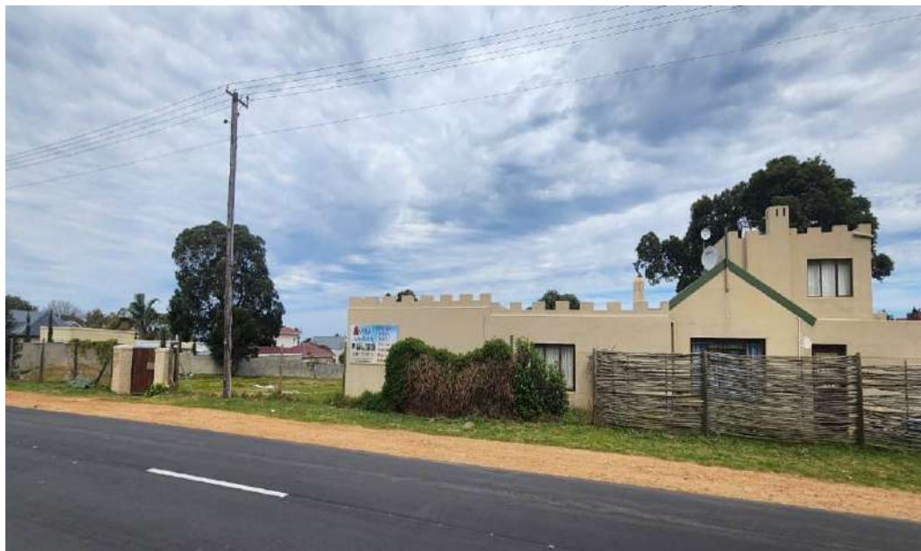
View onto existing dwelling from Main Road
