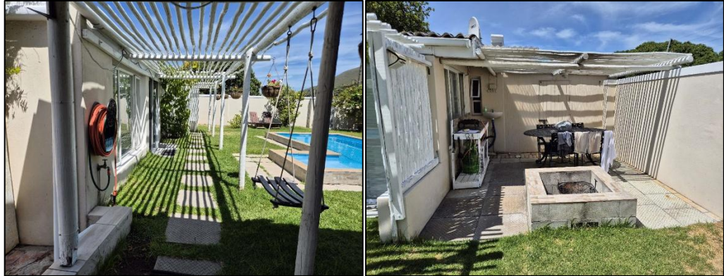
Figure 10: Photographs of the structures exceeding building lines
