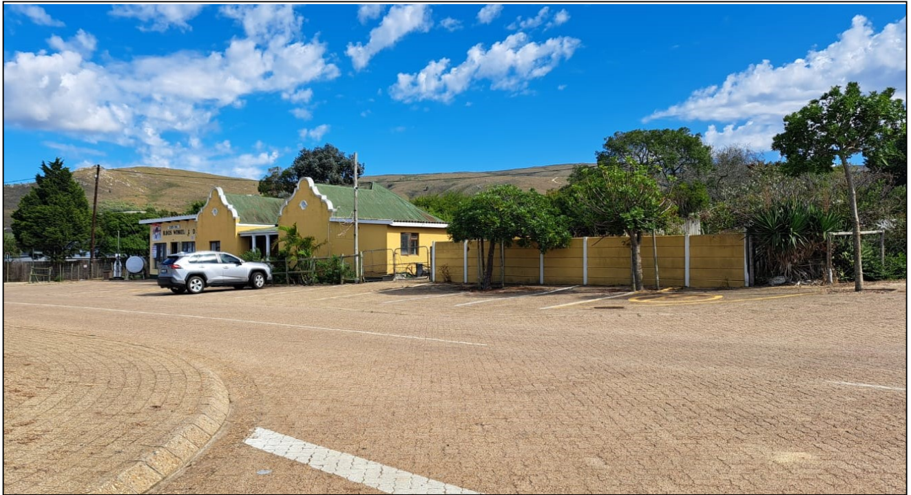
Photo towards the north of the existing shop and liquor store.
