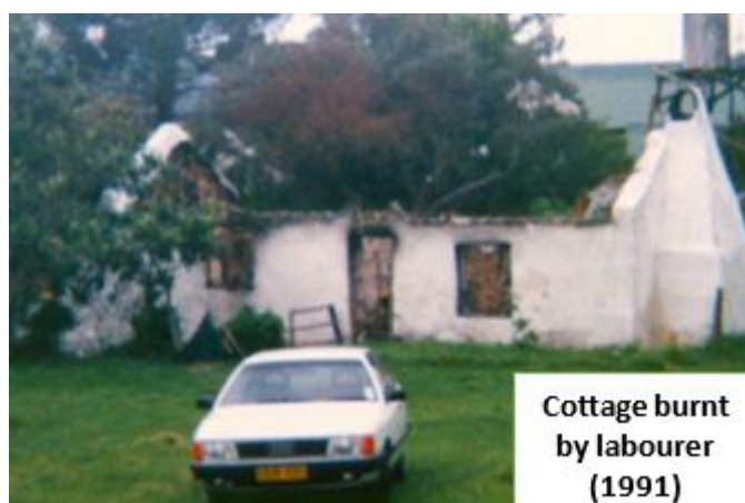
Figure 5: Cottage Following Fire by Labourer (1991) — Portion 16, Farm Rocklands No. 633
