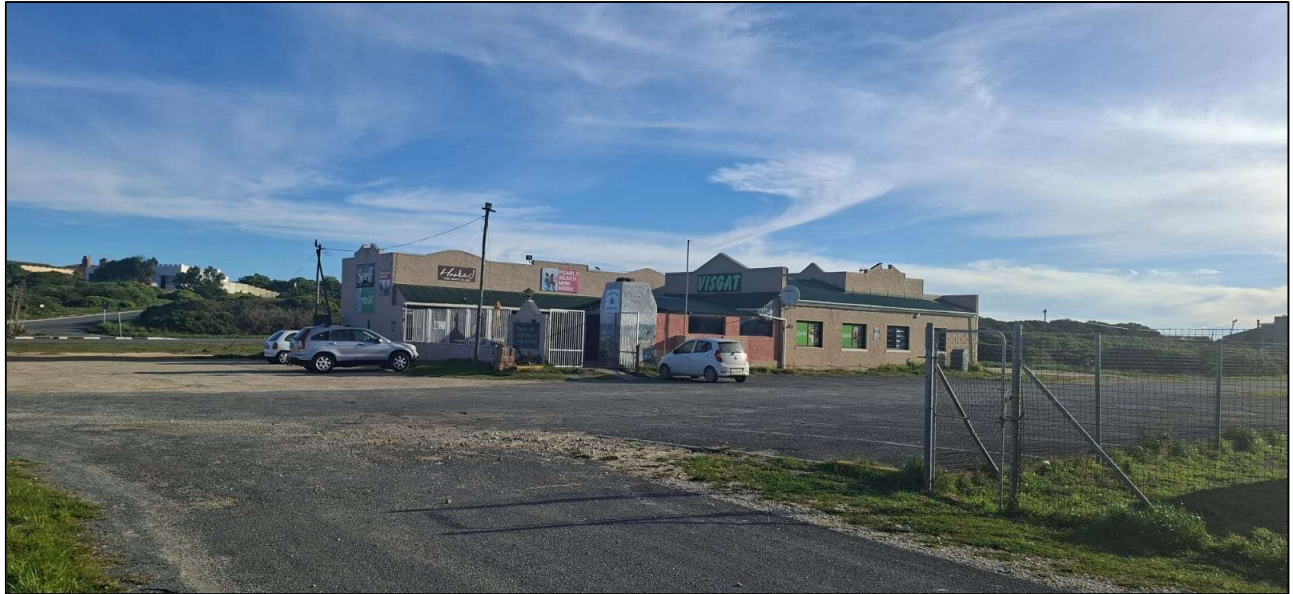
View towards the west
