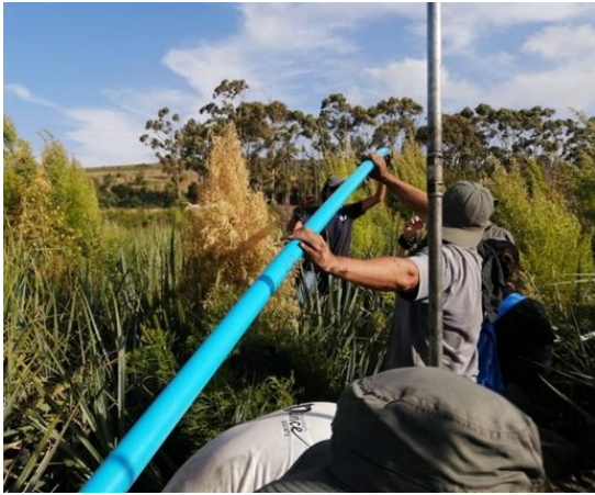
Monitoring wells being installed.
