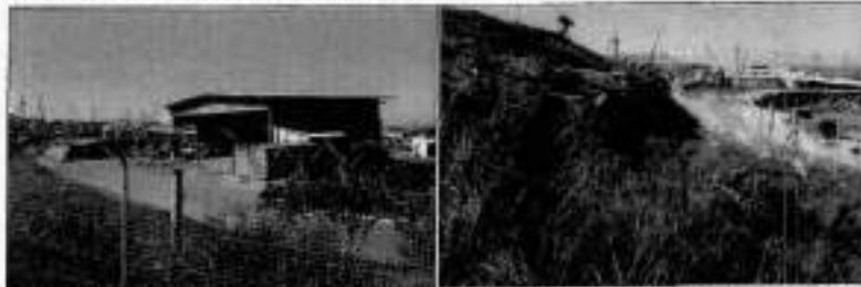
Figure 6: (Left) Waste disposal sorting facility located within the eastern portion of the site; (Right) Excavated channel which has been stabilised by means of a gabion wall, located to the north of the sorting facility.
