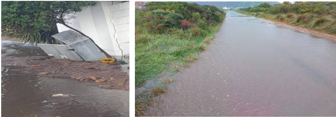
Figure 16: Damages Flooding Pringle Bay
