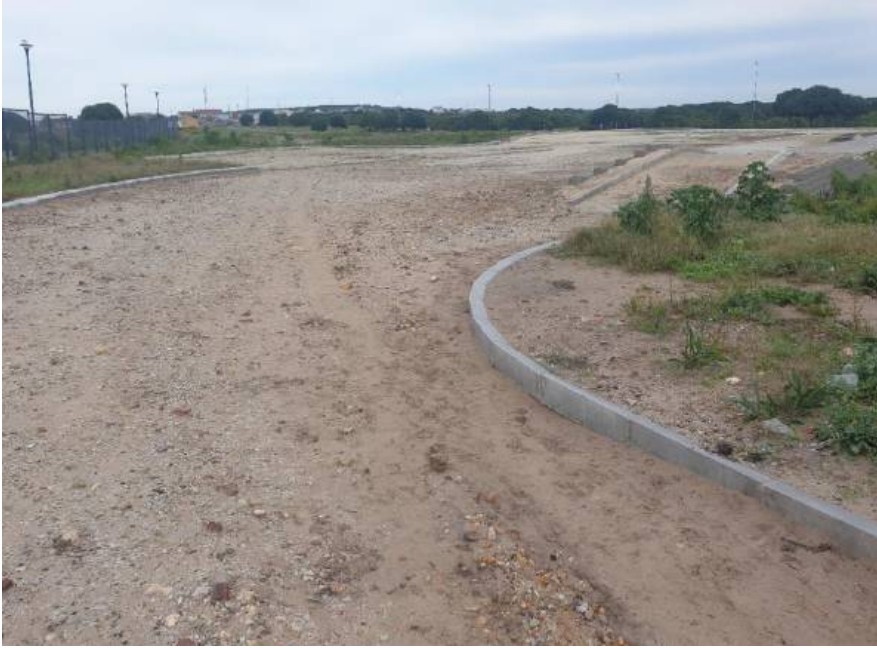
Figure 18: REPAIR DAMAGED SURFACE AND LAYERWORKS
