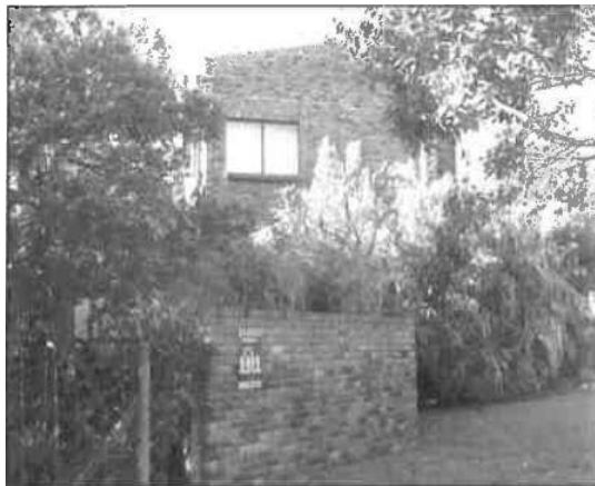
Fig 2 Corner west wall and north fence
