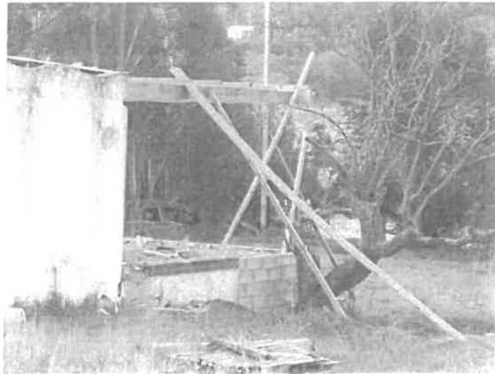
Second dwelling – rebuilding on 26 March 2025
