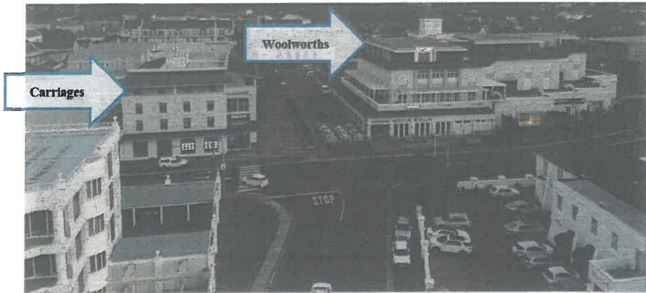
Figure A6: Street view showing the Carriages (Erf 848 Hermanus) on the left (excluding proposed penthouse) and Station Square (Woolworths Building) on the right.
