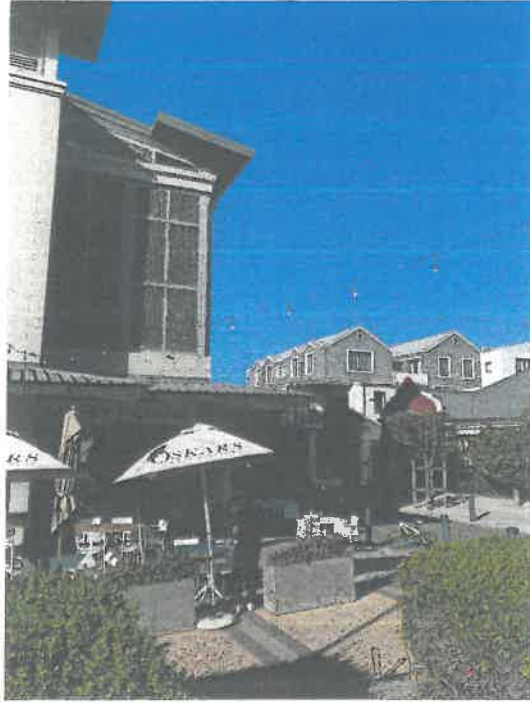
Figure A2: High Street view – Carriages on Erf 848 Hermanus(left) and Marine Square (right, background), illustrating clear spatial separation.
