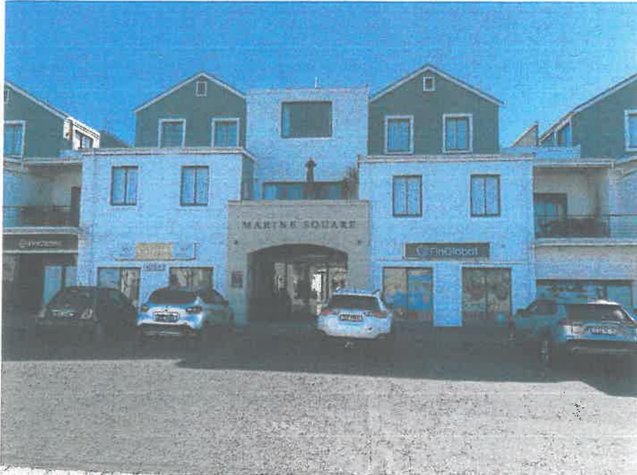
Figure A4: Marine Square's south western façade – demonstrating 3 storey, courtyard design facing an internal street.
