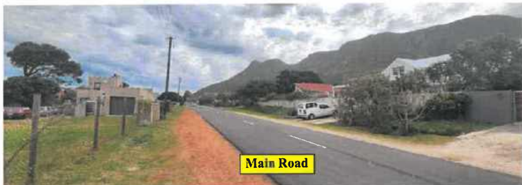
Main Road from east to west with subject property on the left
