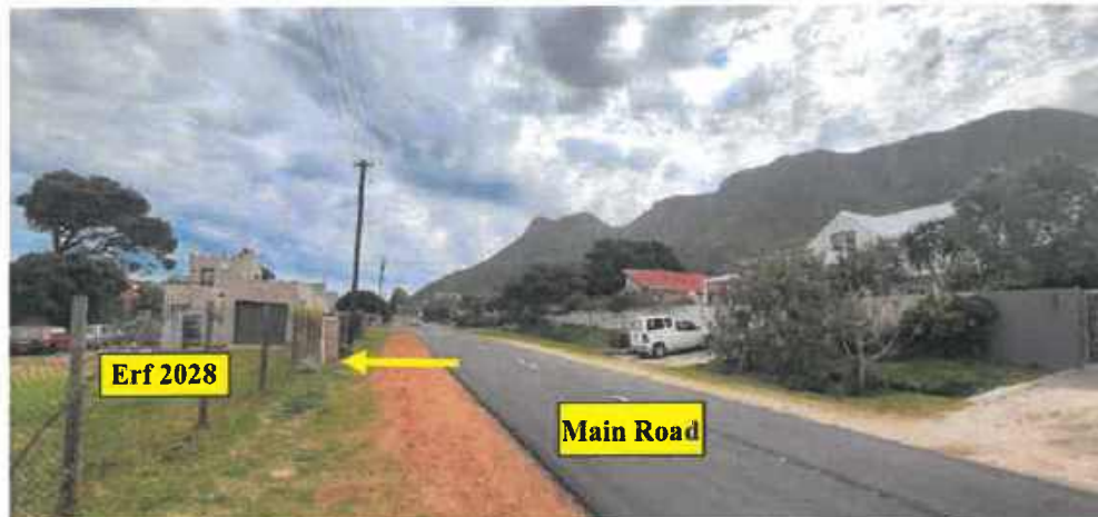
View along Main Road with subject property to the left and existing entrance
