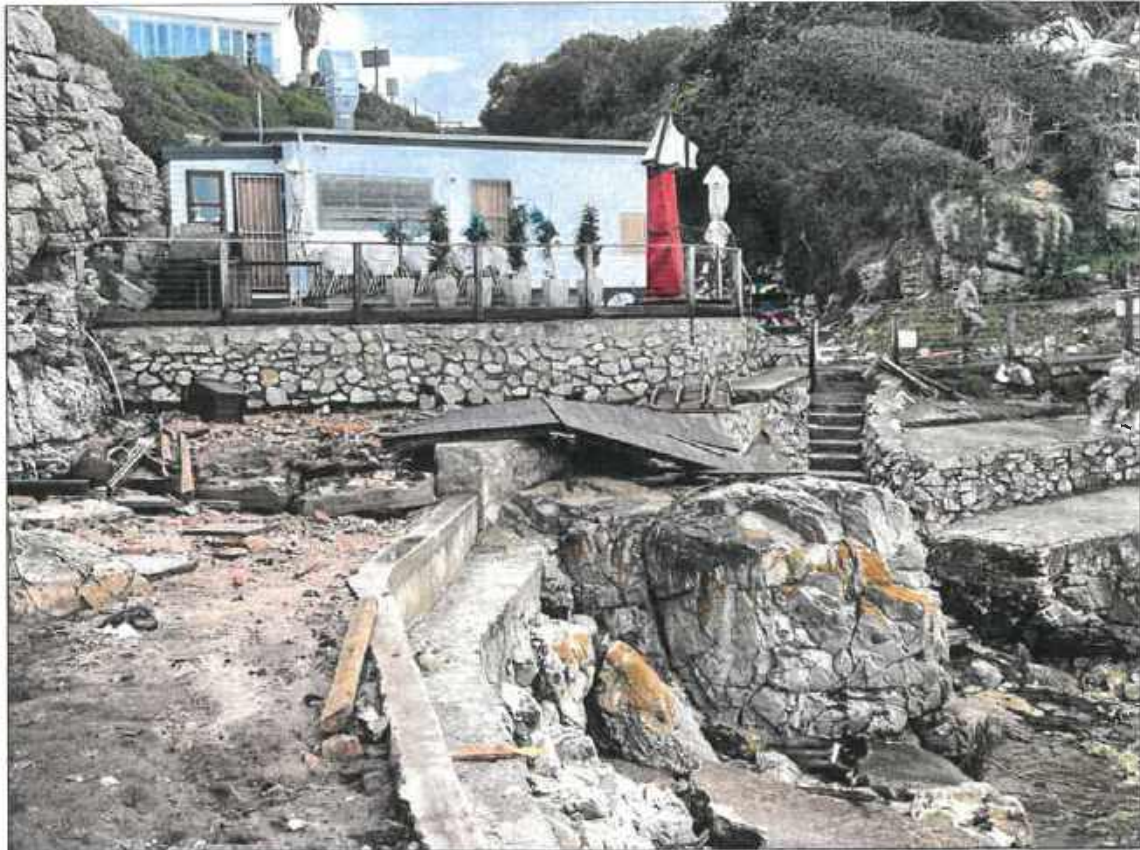
(Figure 2 depicting the damage of the September 2023 storm event with the wooden decks, furniture and balustrade completely destroyed)
