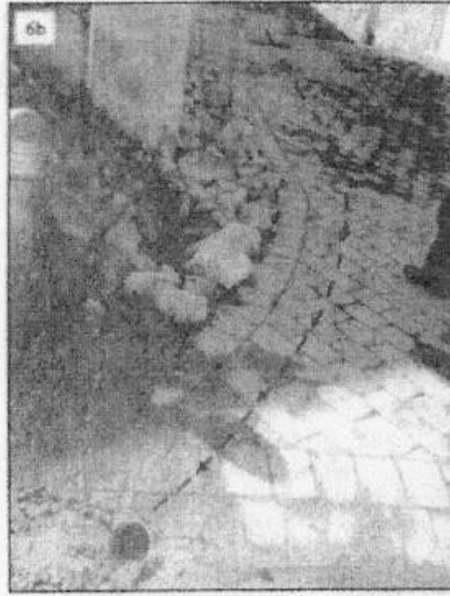
Subsoil drain outlet, which used to dispose seepage water at the surface where the turning circle and driveway merge.
