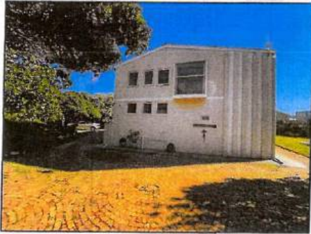
Photo 3: Eastern View (from Priestley Road)
