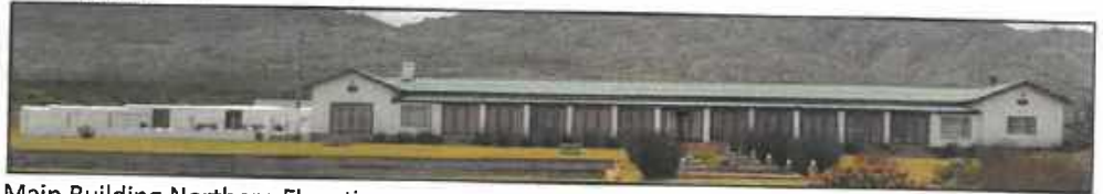
Main Building Northern Elevation
