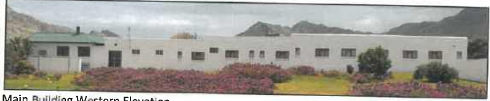
Main Building Western Elevation
