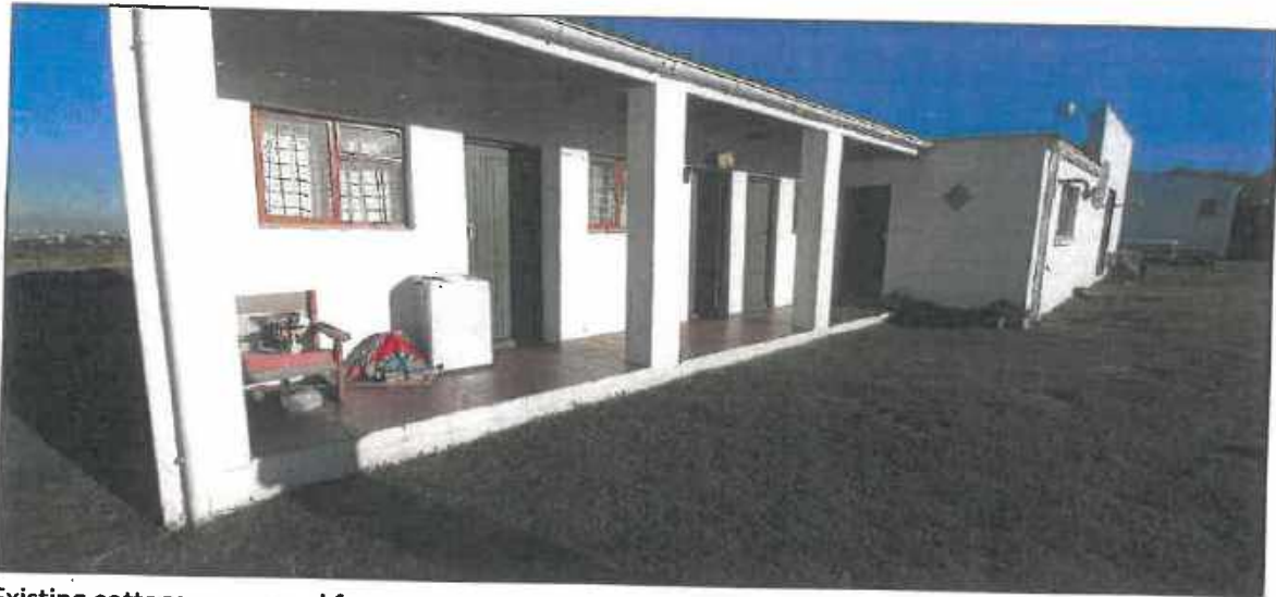
Existing cottages proposed for expansion. No natural vegetation present.
