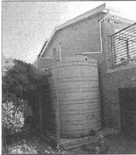
Image taken of tanks on Erf 338
