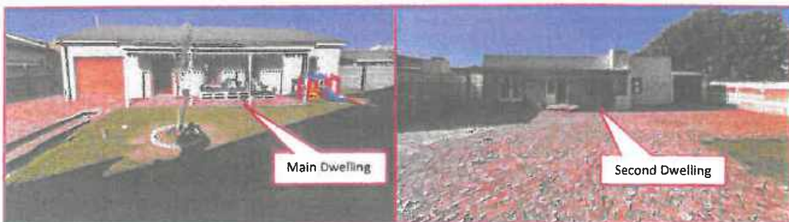
Figure 6: Front View of Main & Second Dwelling
