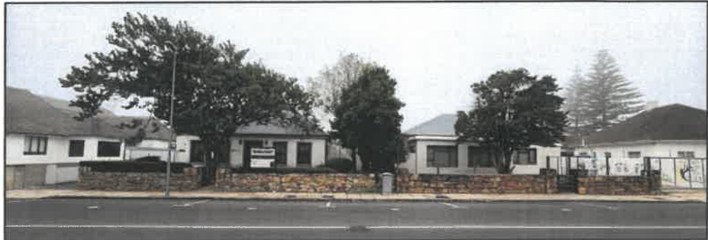
Figure 11: Photograph from the road
