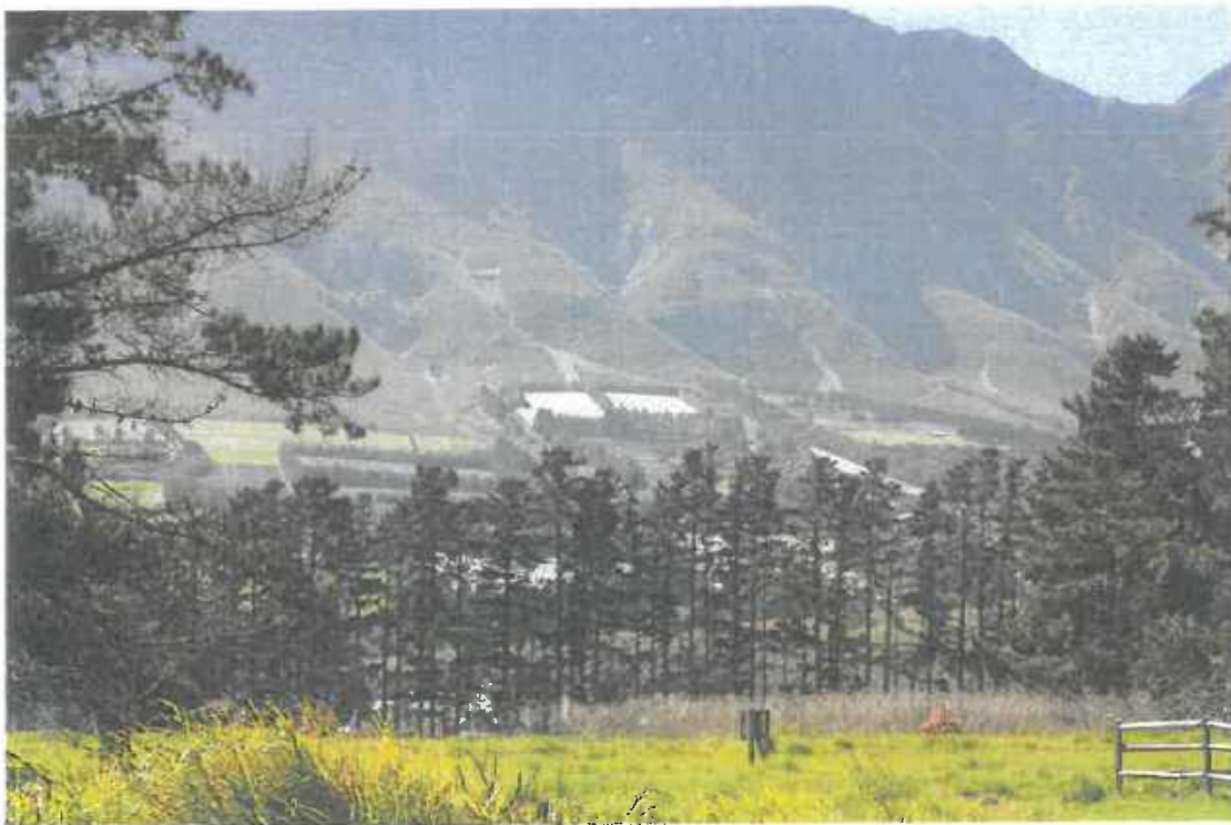
Image S: The tunnels can easily be seen from Four Seasons Stud farm. Despite the row of trees screening the tunnels, they are still highly visible through the trees.
